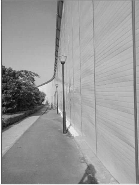
Seal Up Site Hoarding Base To Prevent Water Seepage To External Public Footpath
