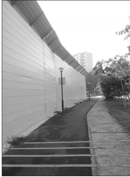
Seal Up Site Hoarding Base To Prevent Water Seepage To External Public Footpath
