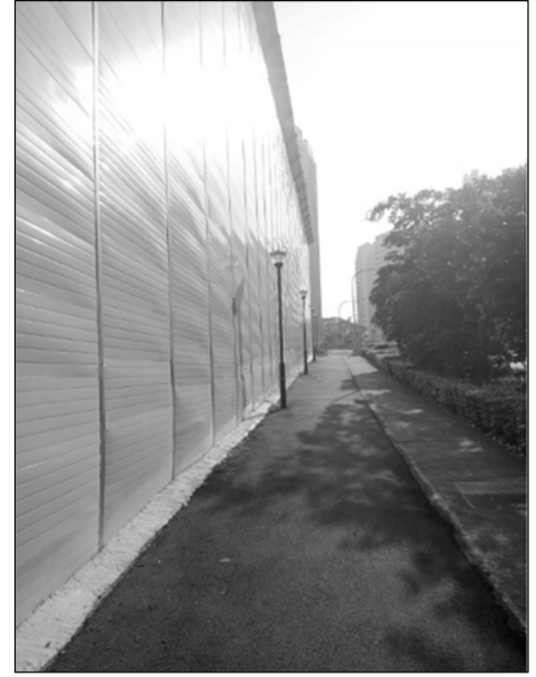
Seal Up Site Hoarding Base To Prevent Water Seepage To External Public Footpath
